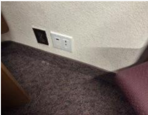
Camera Run should run to the side where these are found.
